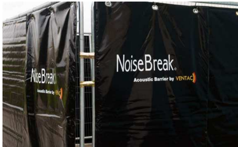
Figure 10.8: Temporary Construction Noise Barrier © Ventac
